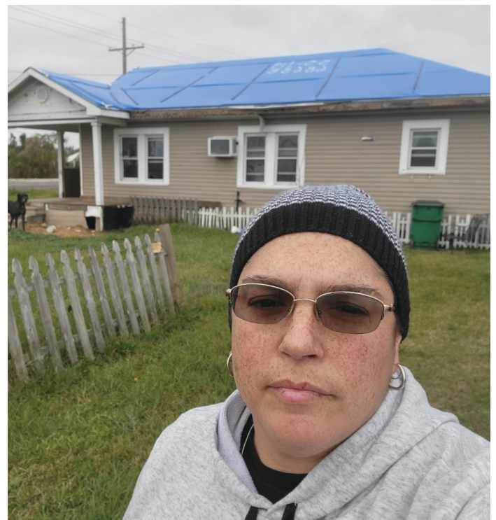
Michelle Rae-Thibodaux Parfait outside her damaged home. Photo courtesy of Michelle Rae-Thibodaux Parfait.
