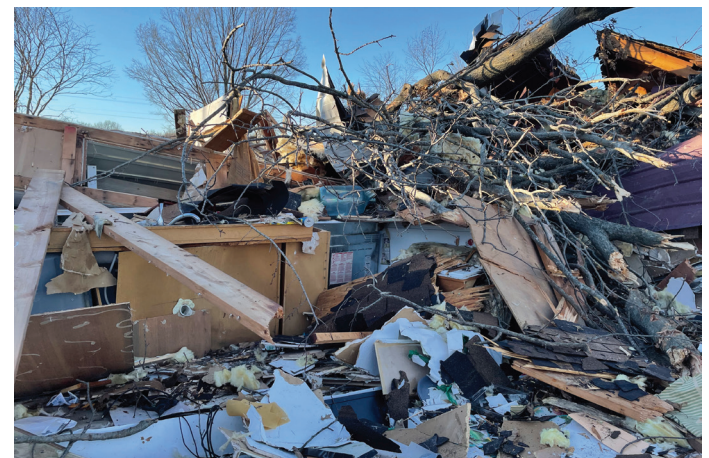
Keith Cardwell, pictured above, and his family lost their home to the December tornadoes. Photo courtesy of Keith Cardwell
