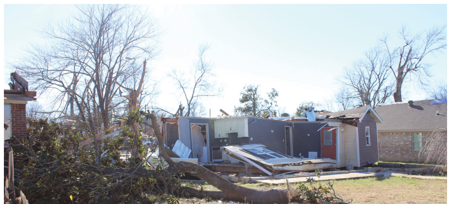
Tornadoes tore apart this Arkansas home. Housing remains one of the most common barriers to recovery. The Red Cross is working with local nonprofits to help residents overcome these barriers and find permanent housing solutions. Photo courtesy American Red Cross of Missouri and Arkansas
