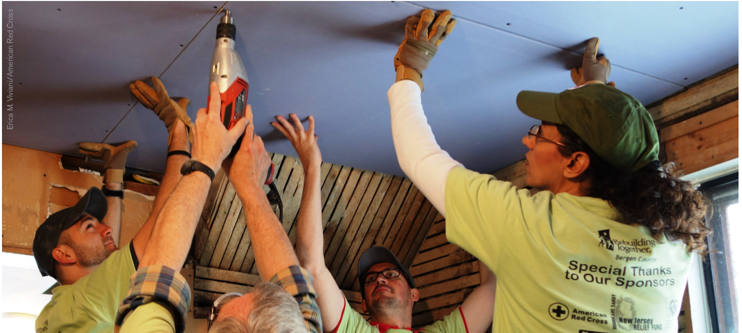
Red Crossers hang drywall at a Bergen County, N.J., home damaged by Superstorm Sandy, as part of Rebuilding Together's National Rebuilding Month.
