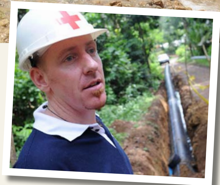
TOP: Boys play in water that has travelled through a 20-mile pipeline built by the American Red Cross in Calang, Indonesia. ABOVE: Kelvin Shingles, an American Red Cross water and sanitation delegate, explains how this pipeline will bring water to thousands of people in Galle, Sri Lanka, where many resettlement houses have been constructed.
